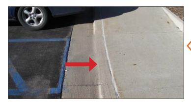
**SOLUTION:** Clean large cracks and fill them with appropriate caulking material. In some cases, rope caulking may be necessary to use as a base to keep the filler material in place.
