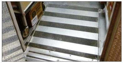
**SOLUTION**: Install traction strips on the walking surfaces of ramps, or apply another slip-resistant treatment such as lacquer and mineral aggregate. Consider installing slip-resistant resin ramps when planning new ramp construction.
