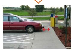
**SOLUTION:** Repair or replace concrete to provide a smooth transition between sections. Grinding and mudjacking are typically more economical than replacement.
