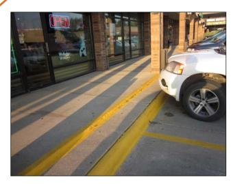
**PROBLEM:** Gaps between sidewalk sections can catch heels, creating a tripping hazard. In addition, large gaps collect water, which can aggravate frost heaving.
