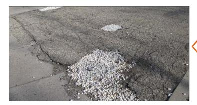
**SOLUTION:** Perform routine inspections and repair potholes as soon as possible. Gravel may be added as a temporary solution until more permanent repairs can be made.
