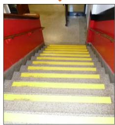
**SOLUTION:** Repair or replace deteriorated stairs. Slip-resistant tread covers can easily be retrofitted to existing stairs.
